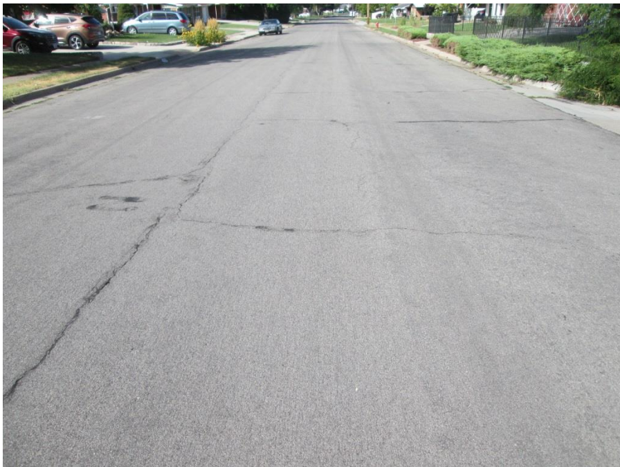
Photo 2. Good Surface Drainage – 350 South from 200 West to 250 West
